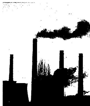
Fig. 5.10 A thermal power plant
