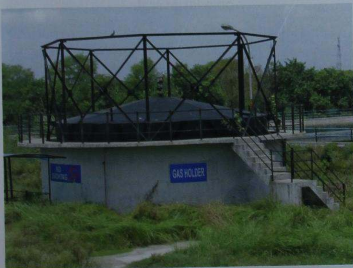
Fig. 5.16 Biogas holder in a sewage treatment plant
