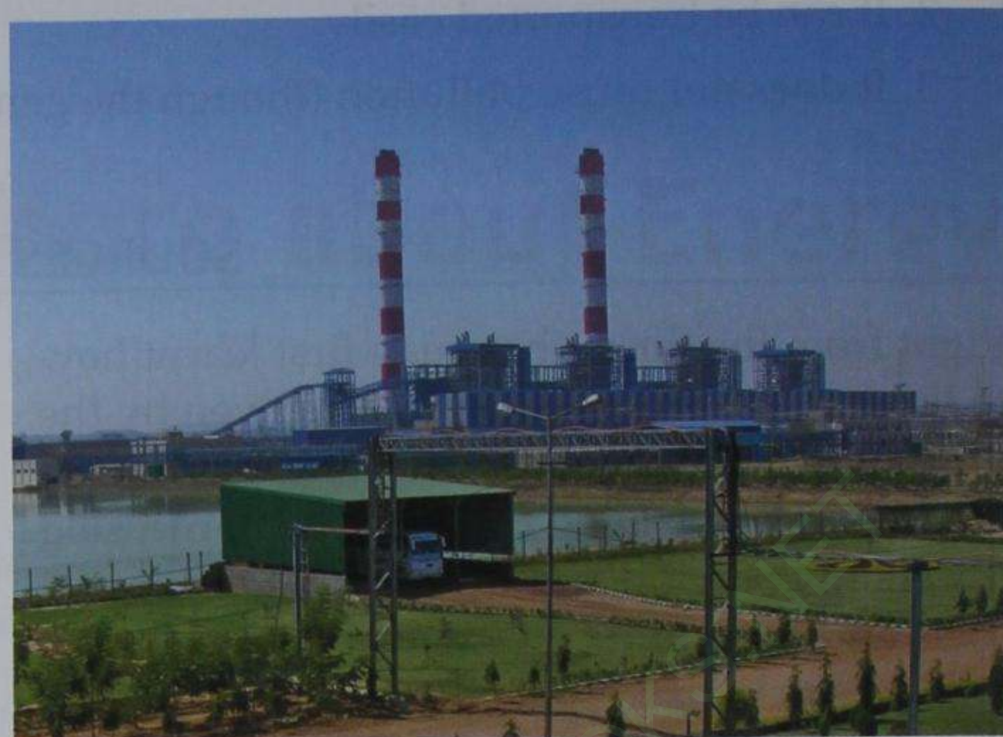
Fig. 5.3 In a thermal power station, fossil fuels are burnt to produce steam, which is used to generate electricity.
