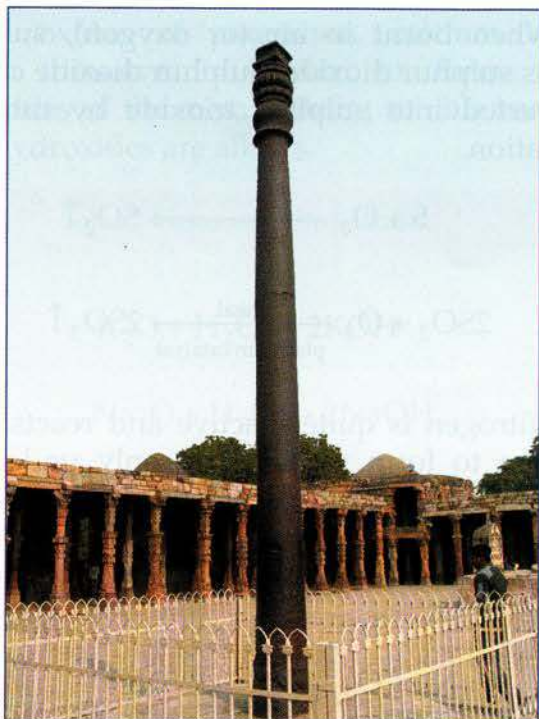
Fig. 6.6 The iron pillar at Delhi has not rusted for centuries.
