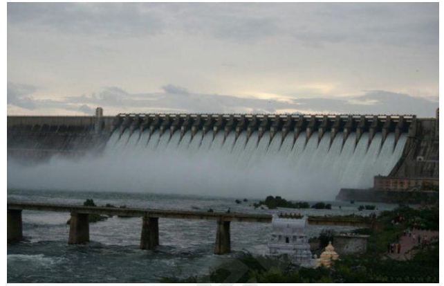
The Hirakud dam helps in controlling floods in the Mahanadi delta and irrigates 75,000sq km of land.
